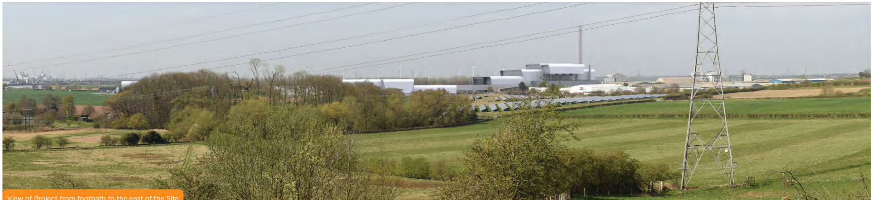
View of Project from footpath to the east of the Site
